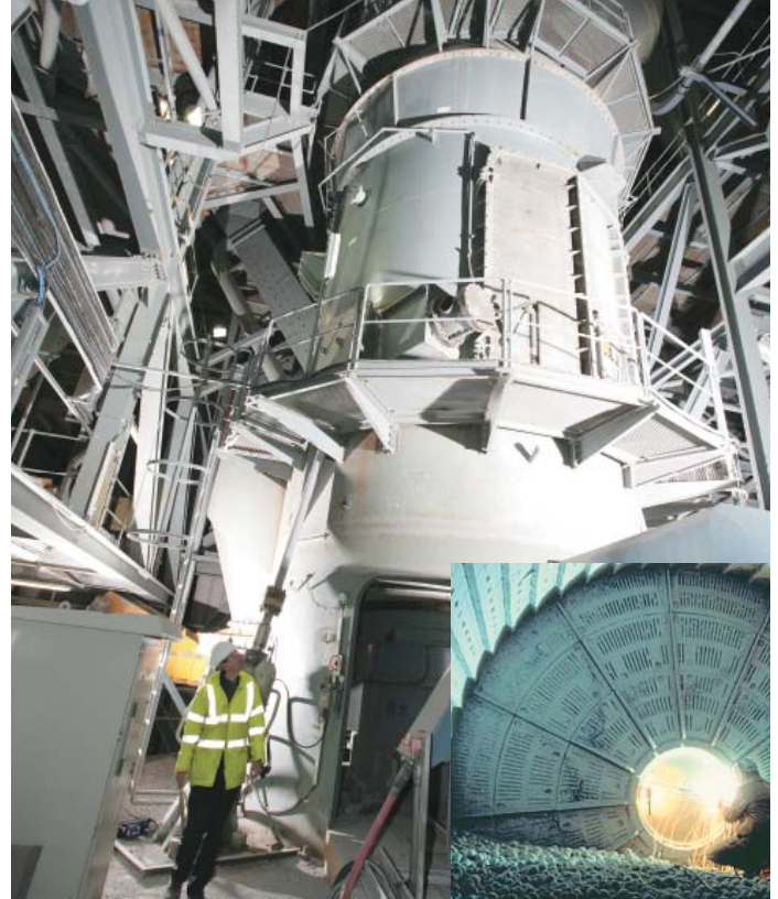
Vertical and horizontal grinders can benefit from the use of ABB drives.
