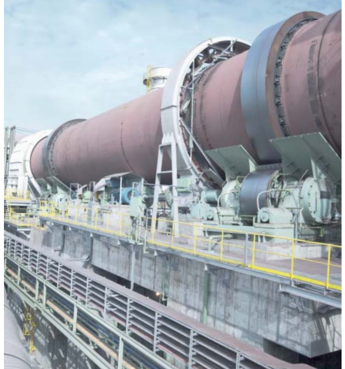
ABB drives' DTC plays an important role in the efficient running of kilns.
