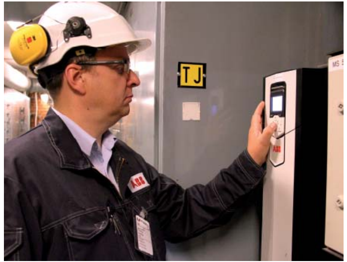
The ACS880-01 wall-mounted industrial drives are easy to use and configure for optimal water pump flow.
